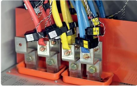
Split core CTs can be installed without having to disconnect critical power systems.
